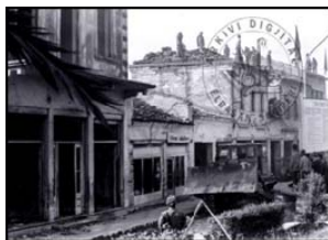
Figure 7: Old Bazaar during Demolition in year 1977. (Elbasan Digital archives)
