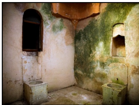
Figure 25: Interior view of bath today (www.panorama.com.al)
