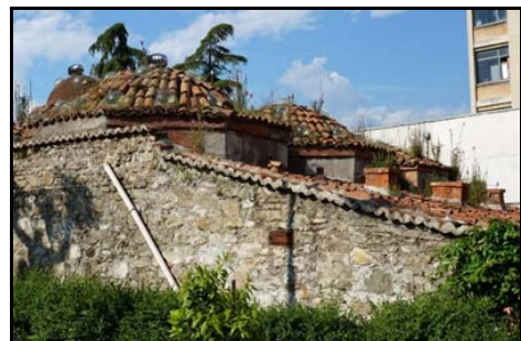
Figure 23: Exterior view of bath. (www.imk.gov.al)
